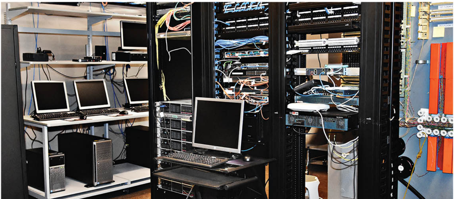
Server Room at Central office Information Technology
